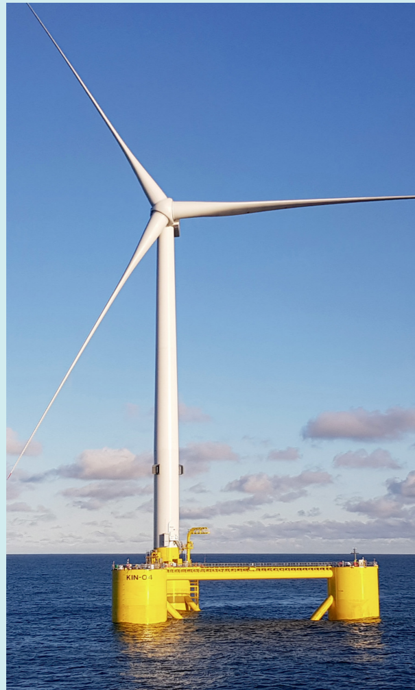
9.5MW Floating Offshore Wind Turbine at Kindardine offshore wind farm (Credit: Principle Power)
