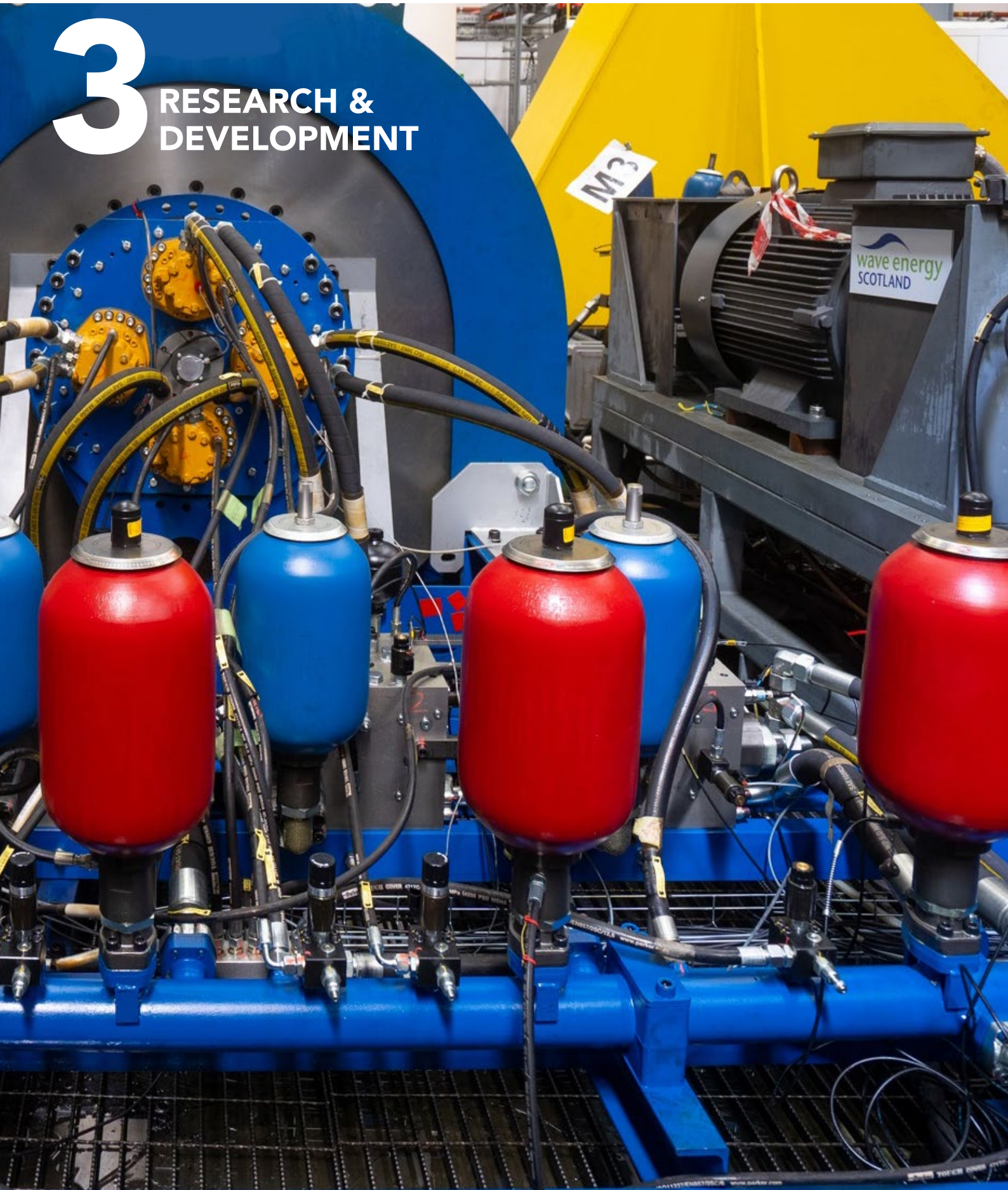
Artemis Intelligent Power's Quantor PTO and test rig (Source: WES)
