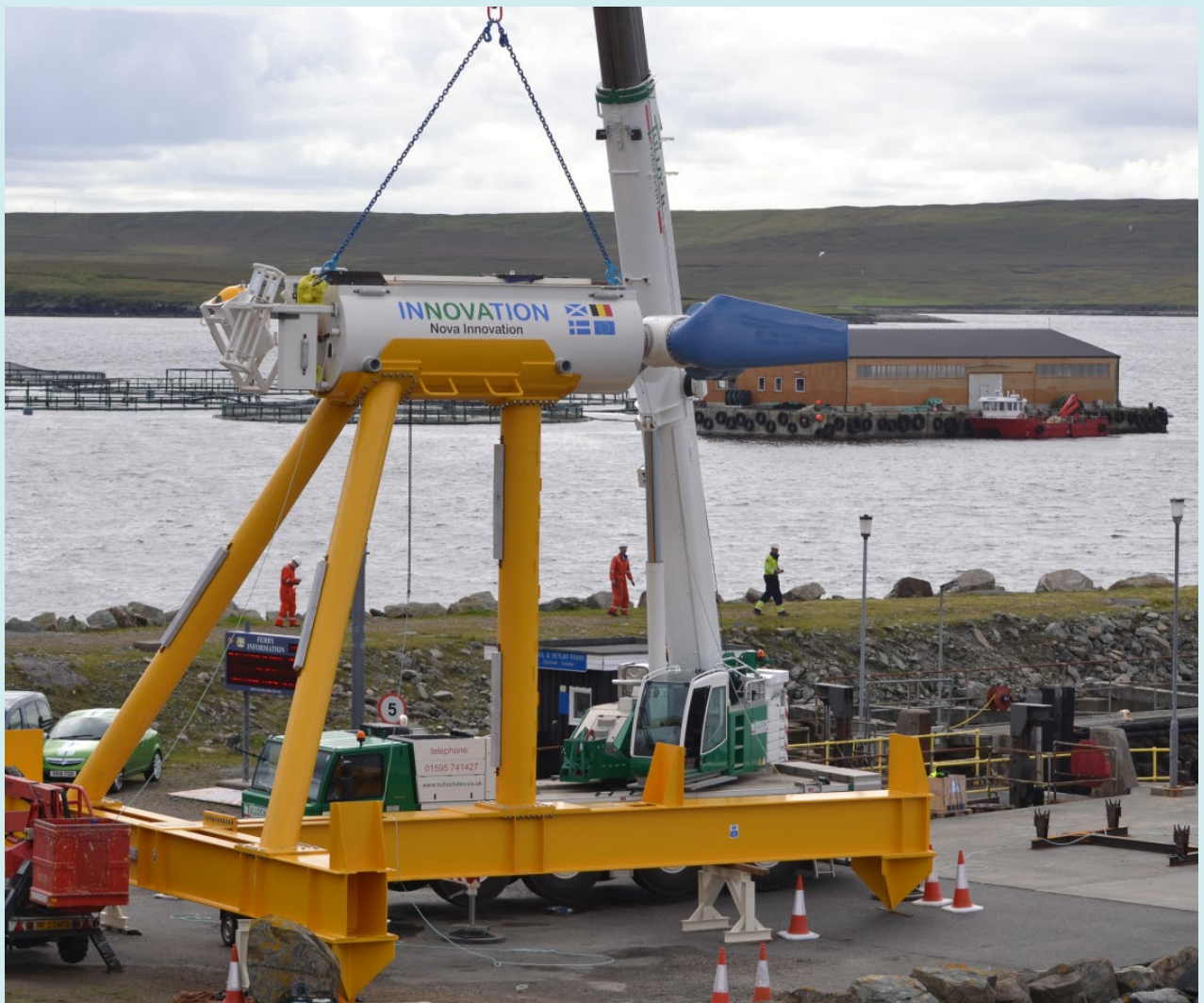
Deploying Nova Innovation Turbine at Bluemull Sound (Source: Nova Innovation)
