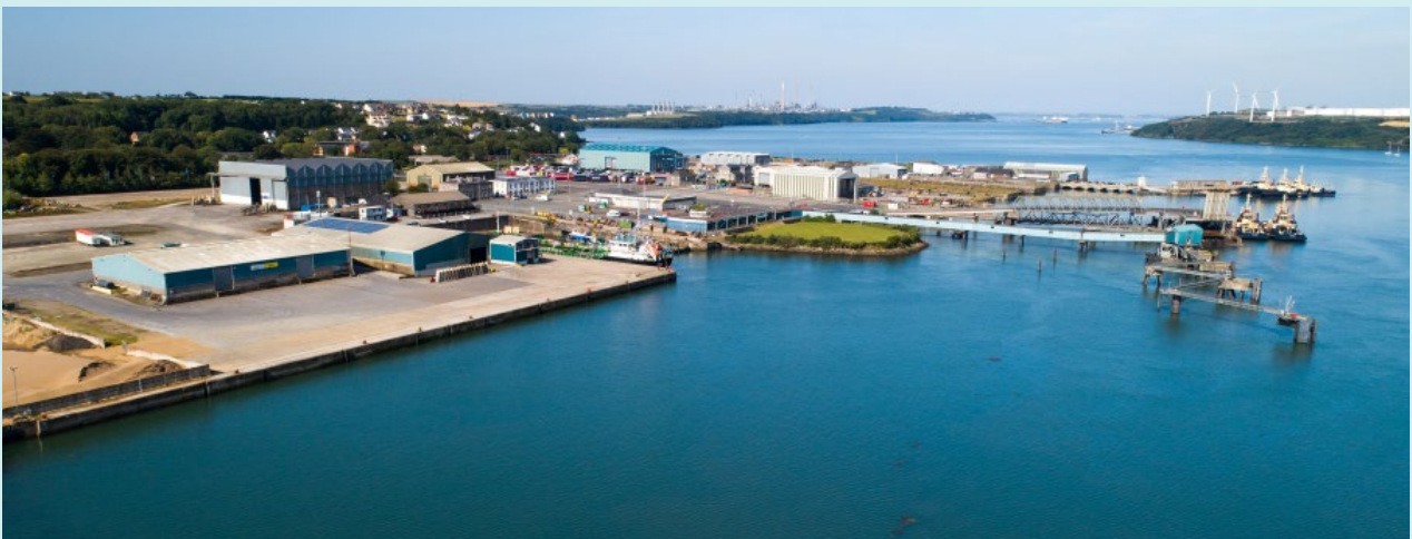
Pembroke port – Phase 1 site (Source: J.Abbott, MEW)
