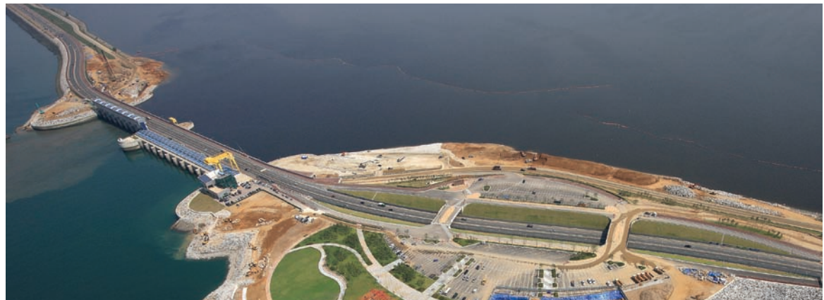
Figure e: Sihwa Lake Tidal Power Station, Korea
