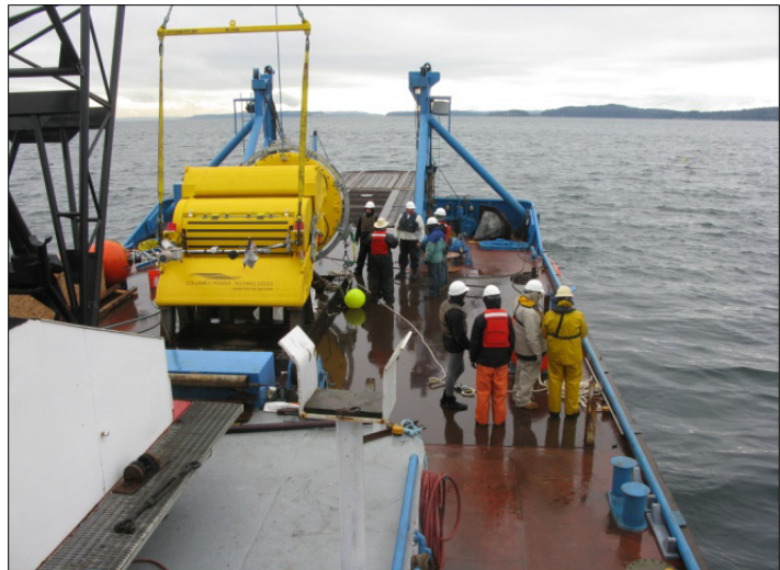
Sound and Sea Technology helps to install Columbia Power Technologies' SeaRay wave energy intermediate scale prototype in the Puget Sound in 2011.
